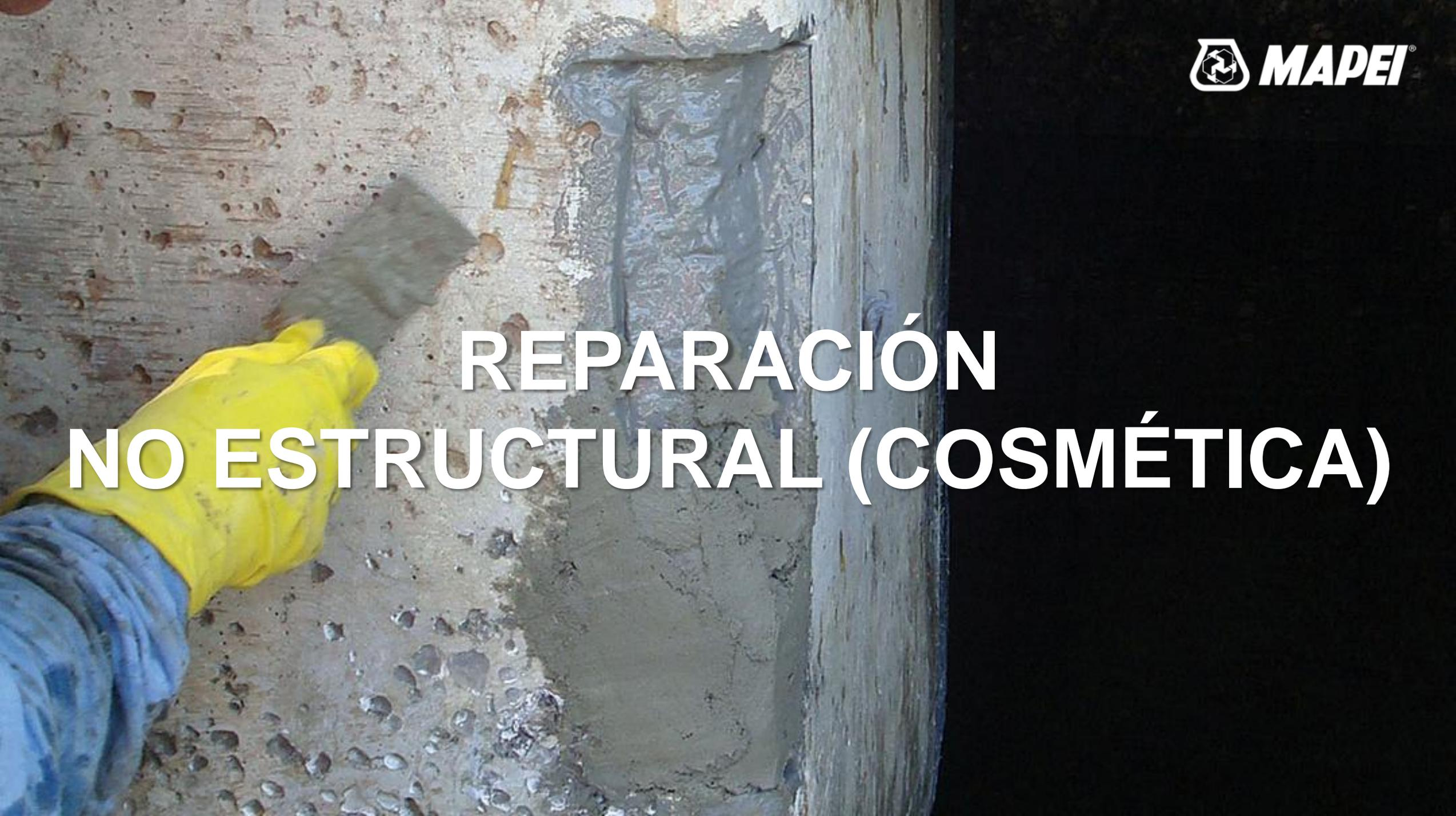
A close-up photograph of a construction worker wearing a yellow glove and a blue sleeve, using a trowel to apply a grey repair material into a rectangular hole in a concrete wall. The surrounding concrete is weathered and stained.
