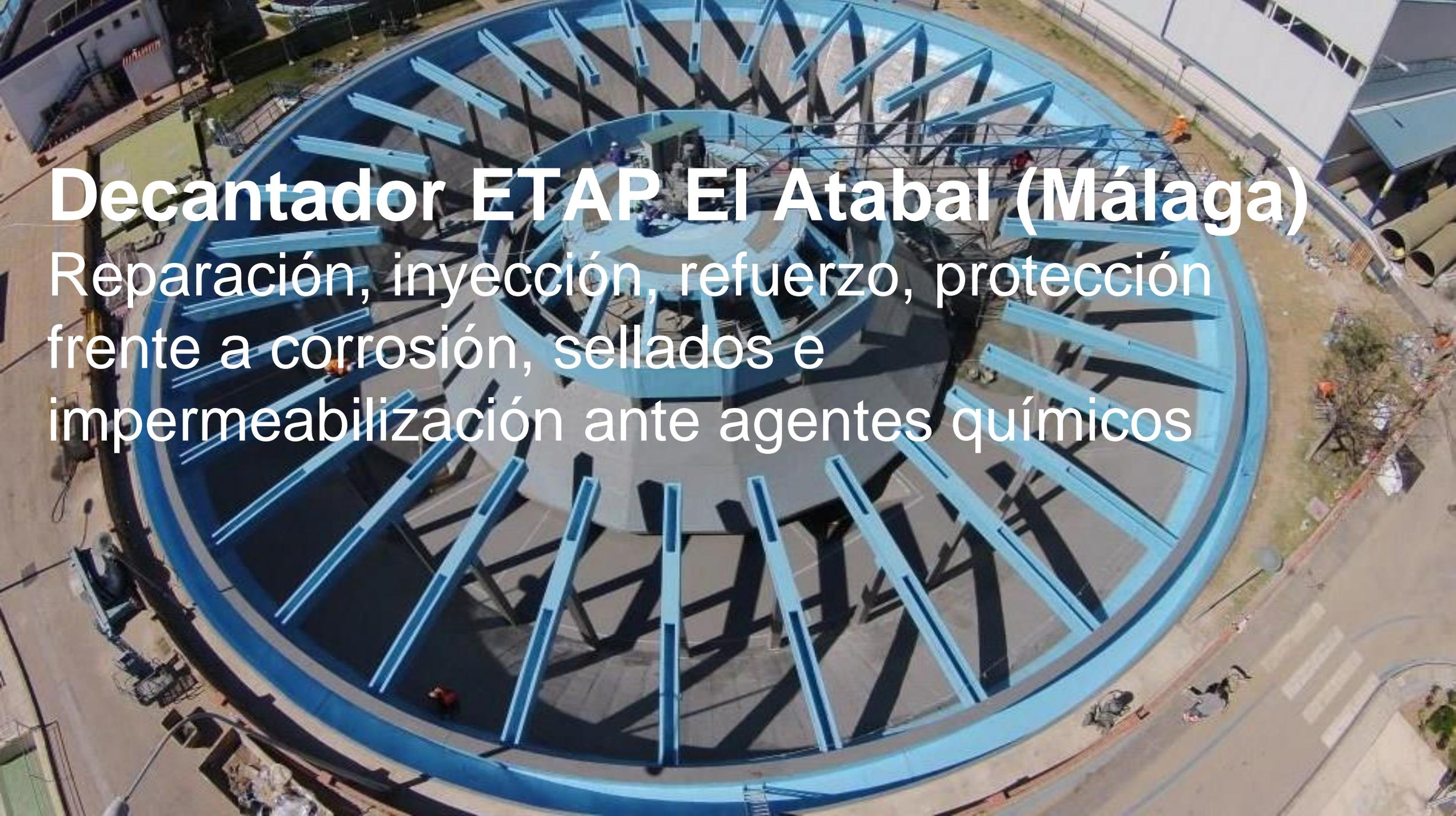
An aerial photograph of a large, circular concrete structure, likely a decantation tank, undergoing renovation. The interior of the tank is reinforced with a dense grid of blue-painted steel beams. Several workers in safety gear are visible on the structure. The surrounding area includes a paved road, some greenery, and industrial buildings.
